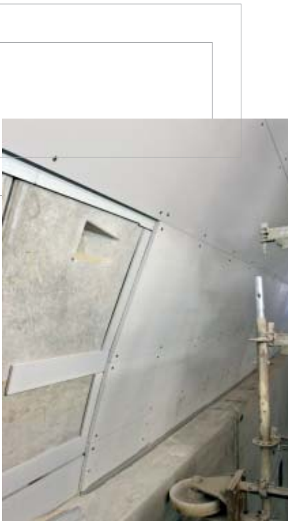
Joint with joint backing strips
