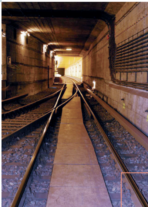
Timber sleeper covering, Berlin underground
