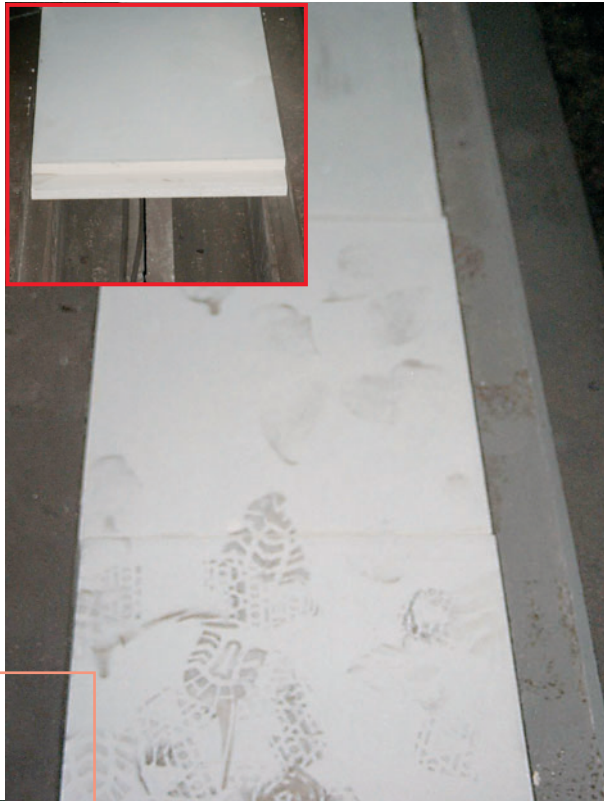
Special solution: concrete trough covering; Munich underground
