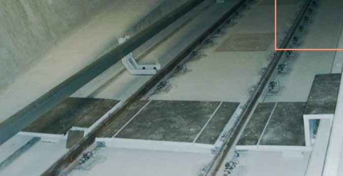
Service alley; Fürth underground
