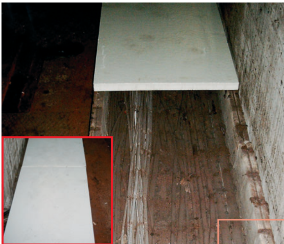
Concrete trough covering; Nuremberg underground
